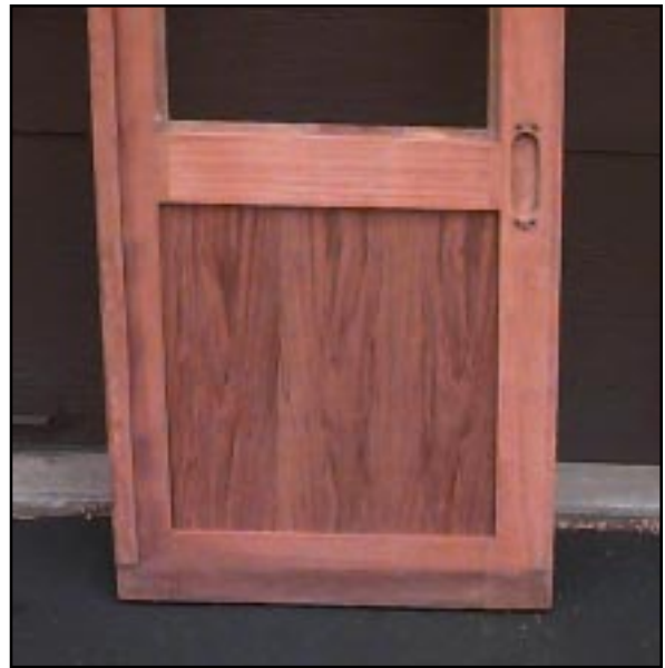
Panel installed, but before molding is attached
