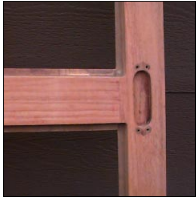
Inside of door with back routed out.
